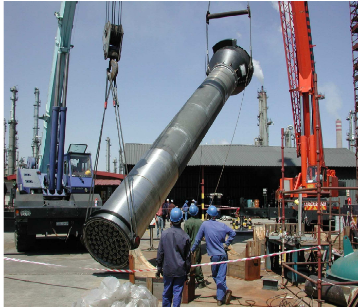
Figure 7. HTER internal being installed
