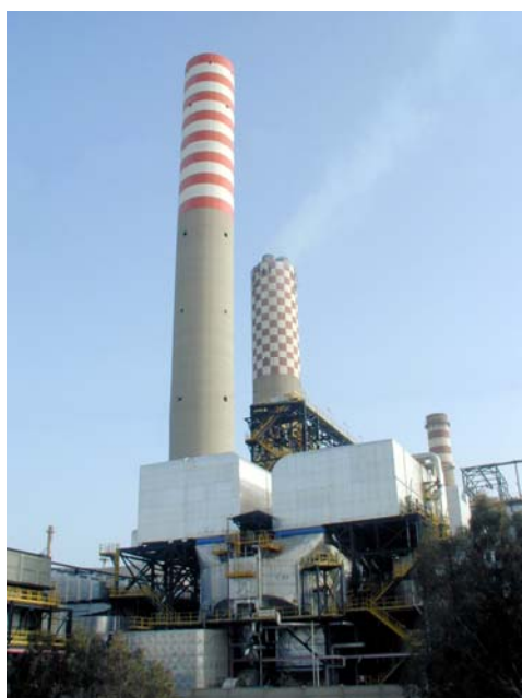
Left: 1,000,000 Nm 3 /h SNOX plant at the power plant of the Agip Petroli SpA refinery in Gela, Italy
