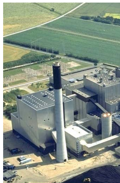
Right: 300 MW coal fired power plant equipped with SNOX at NEFO (Nordjyllands- værket), Denmark
