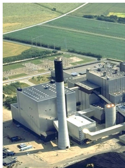
300 MW SNOX™-equipped power plant of Nordjyllandsvaerket, Denmark
