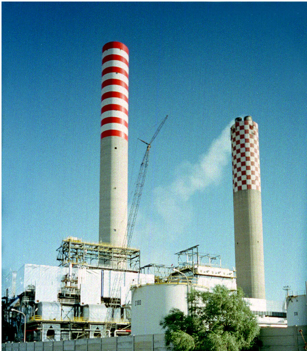
Fig. 2: The SNOX™ plant treating the flue gas from 3 boilers burning high-sulfur petroleum coke at the ENI refinery in Gela, Sicily, Italy. The stack to the left emits 1,000,000 Nm 3 /h of SNOX™ treated flue gas. The stack to the right emits flue gas from the 4th boiler before it was connected to the SNOX™ plant.
