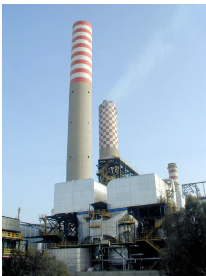
1,200,000 Nm 3 /h SNOX™ plant at the power plant of Raffineria di Gela, Italy
