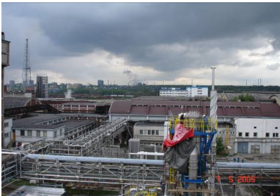
Figure 1: Picture of the BorsodChem MCHZ complex
