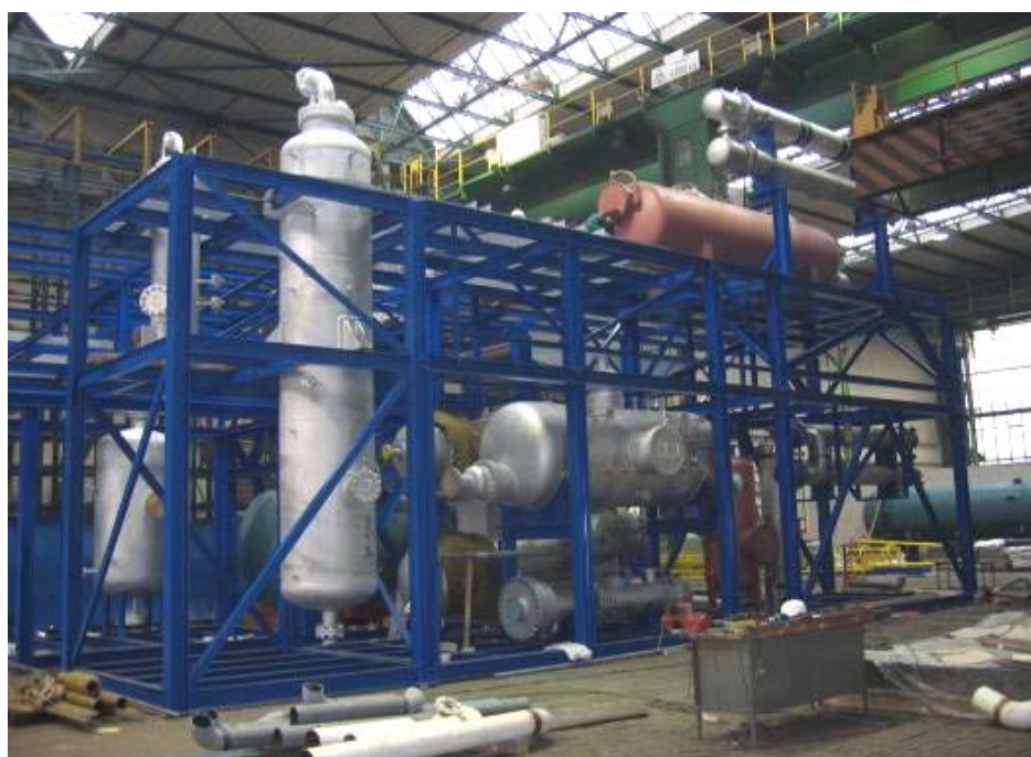
Figure 6: Assembly of HTCR skids in contractor's workshop
