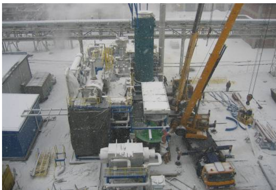
Figure 10: Site installation of skids February 2005
