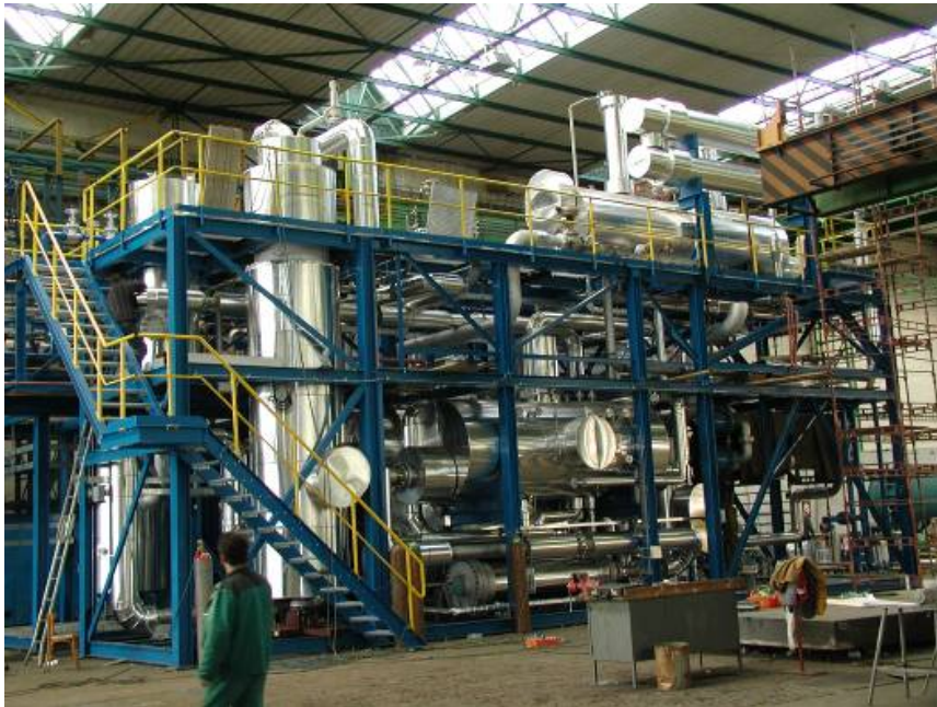
Figure 7: Assembly of HTCR skids in contractor's workshop
