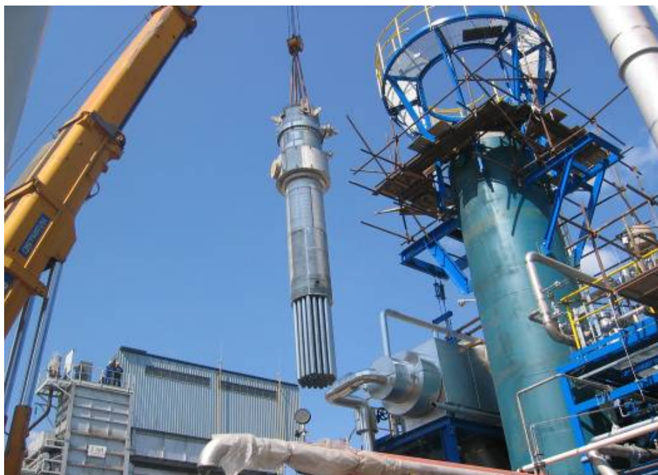
Figure 11: Installation of HTCR tube bundle April 2005
