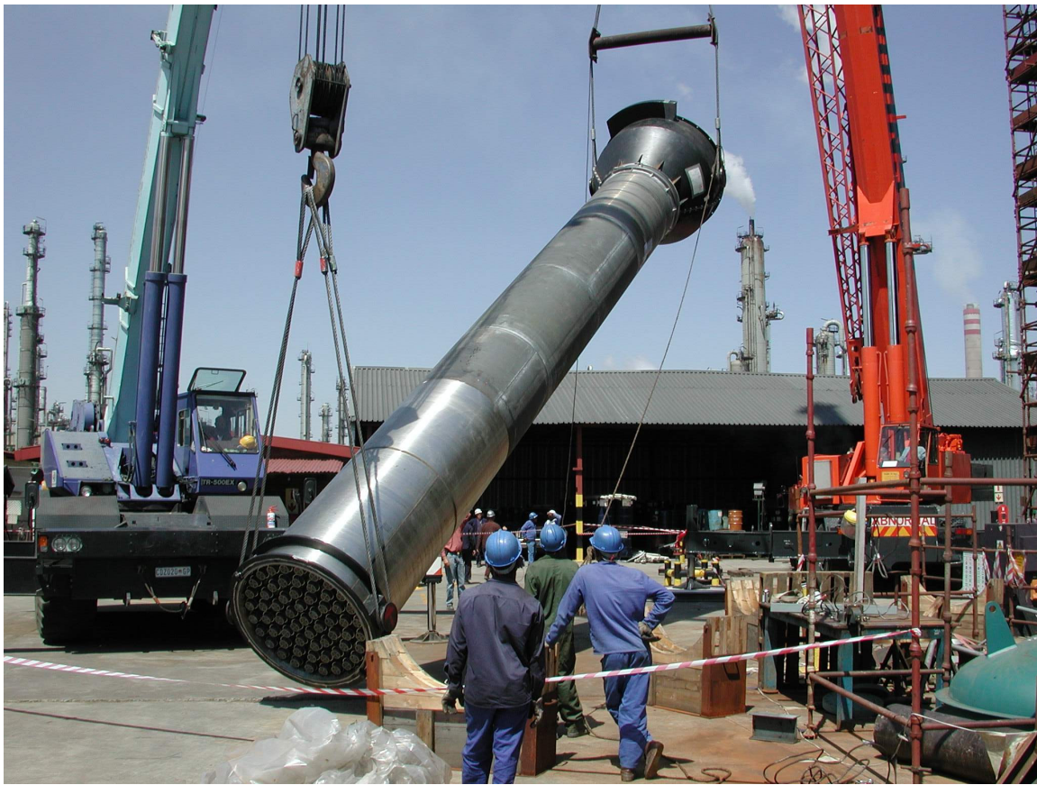
Figure 5: HTER internals being installed
