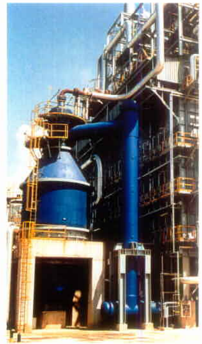
Topsøe CTS Burner for an oxygen-blown autothermal reformer
