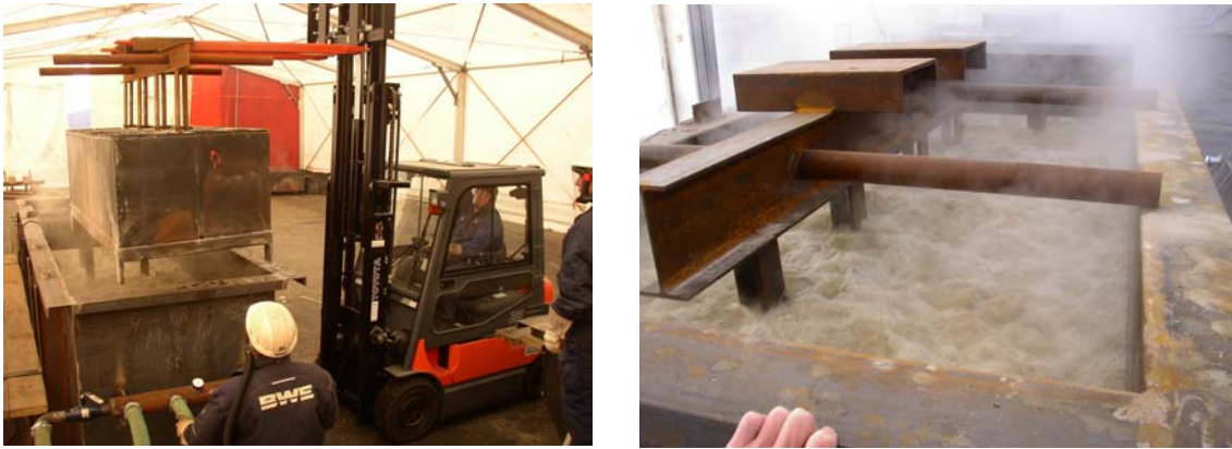
Figure 12 Washing of catalyst modules at Studstrup Power Station
