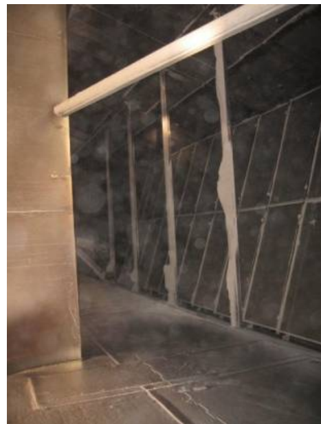
Figure 13 Installation of large particle ash screens in the flue gas duct on Studstrup Power Station Units 3 and 4 (adopted from [8])
